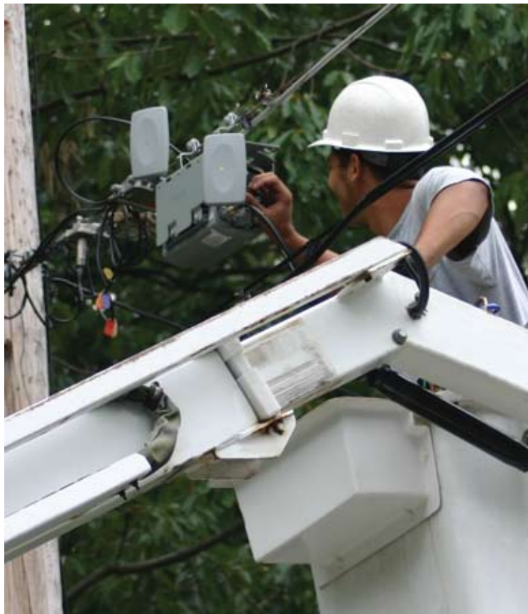
BelAir I00S and BelAir I00SX leverage aerial, pedestal, vault and cabinet stand for mounting, power and backhaul
